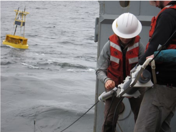
Deploying the Chá Bă mooring. Photo: Diego Sorrentino
